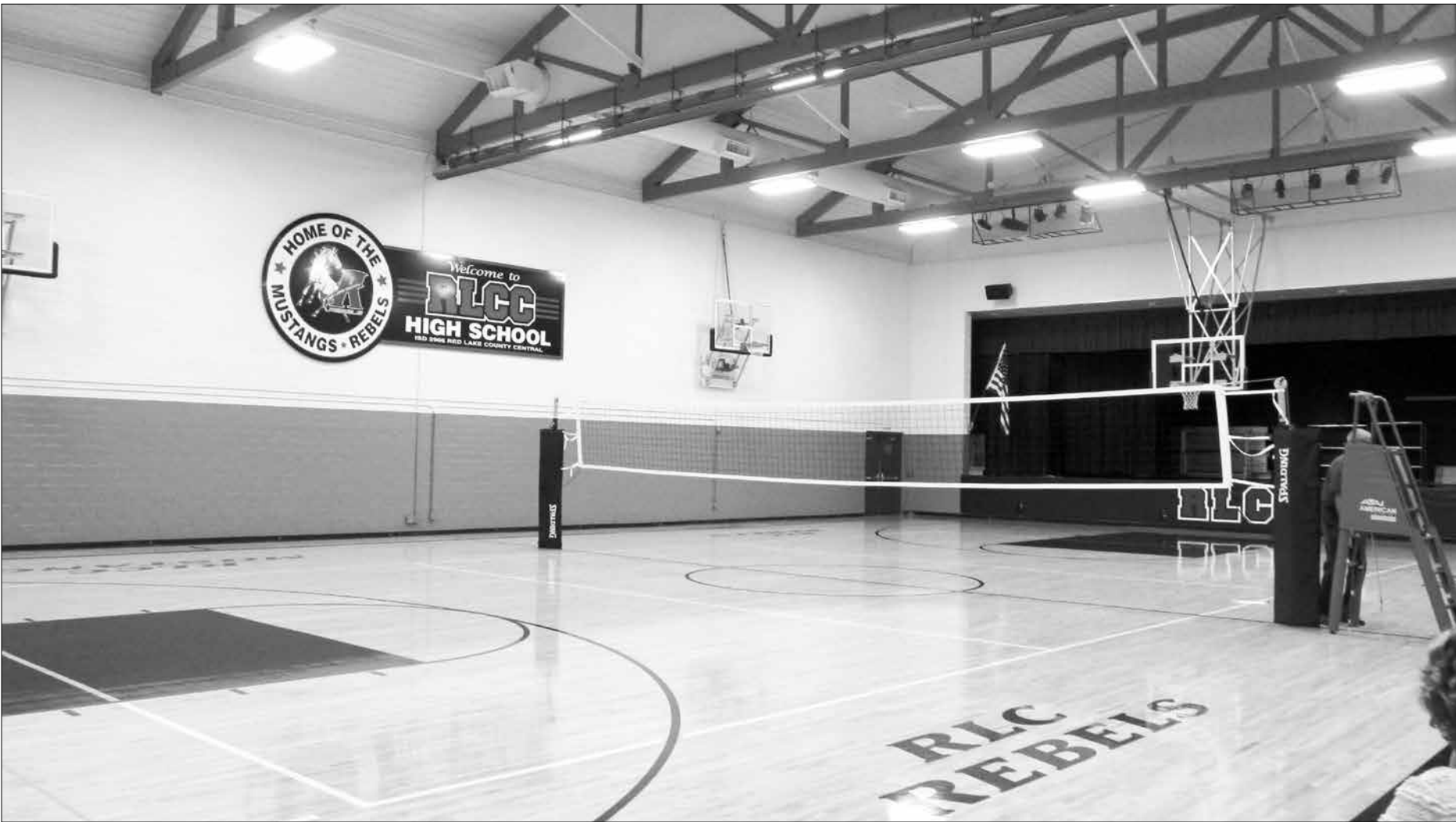
RLCC High School’s gym went through a remodel and new paint job this summer. The ceiling had added insulation and perforated steel to knock down the sound and the walls and some of the stage were painted.
