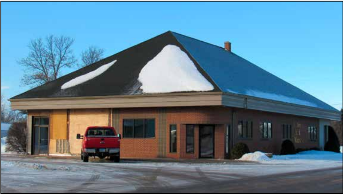
Late Thursday night, the Ultima Bank Minnesota’s Winger branch building was hit by a car driven by an intoxicated driver and sustained substantial damage. The building has been secured and the location is open for business.
