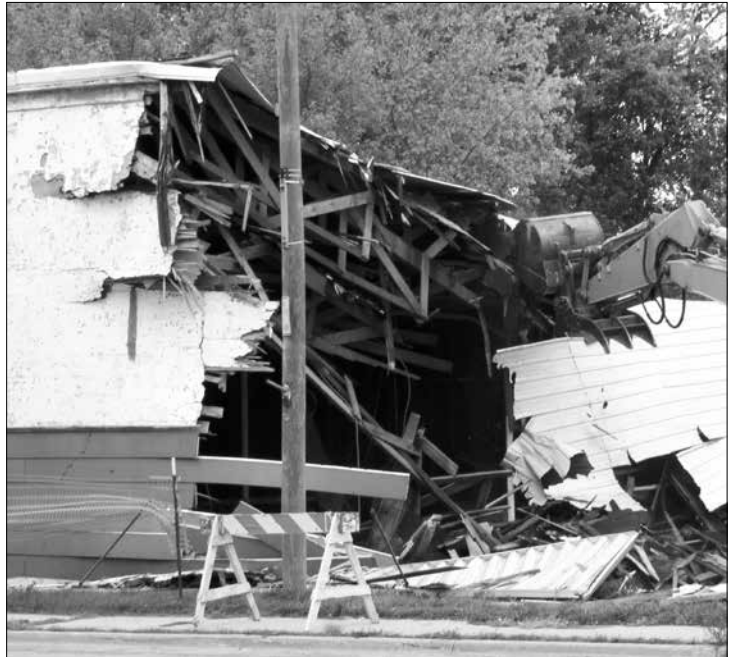
The Helgaas Grocery building was demolished last Monday, September 26, 2016 in Winger.
