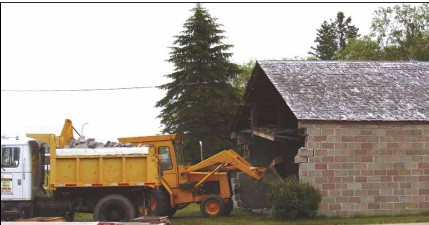
The building at Roholt Park that, in recent years has been used as storage, was taken down on Friday, June 17th. The building had deteriorated over the years and had become a safety issue.
