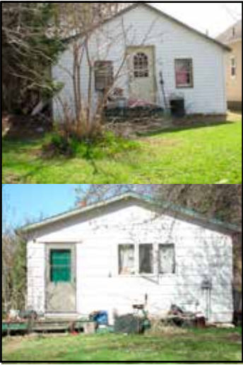
This property in McIntosh has been classified as vacant and a nuisance property. With debris scattered over the yard, it is a hazard.
