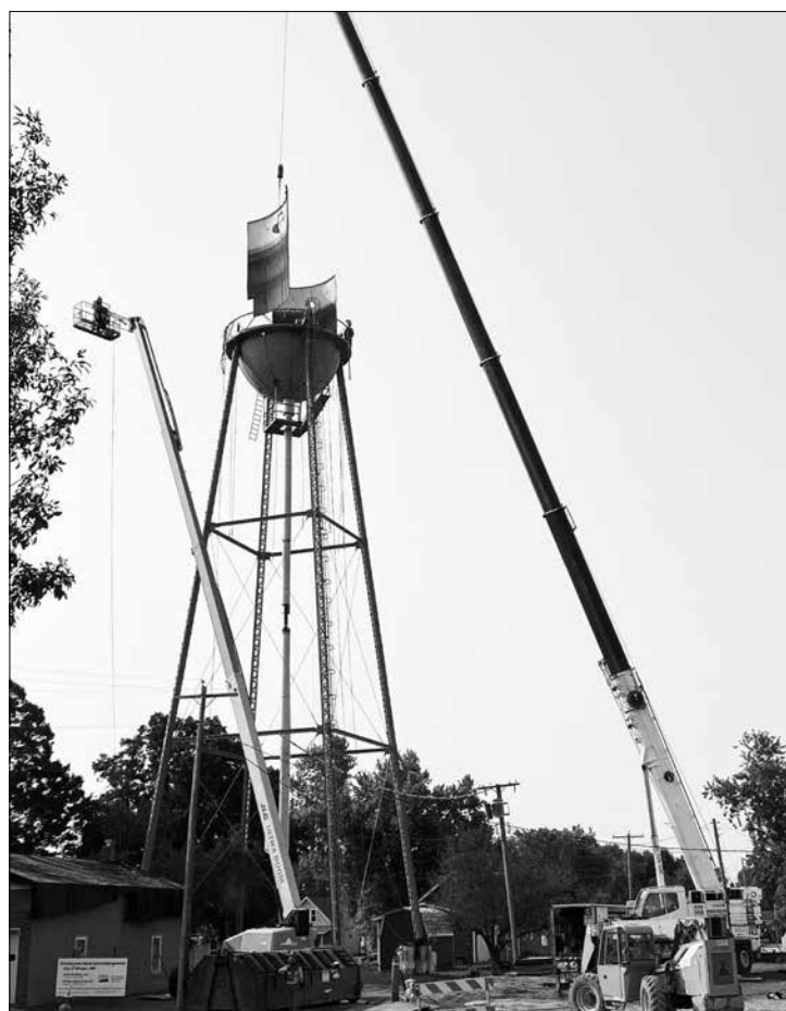
The tank is nearly removed as crews take down the old water tower in Winger last Thursday.
