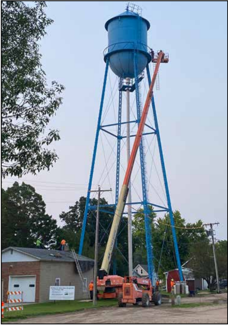
The crews start to take apart the original water tower in Winger, as the entire tower was removed last Thursday.
