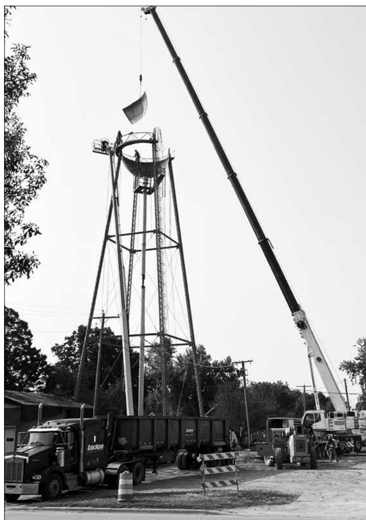
Piece by piece the water tower in Winger was taken down and removed.
