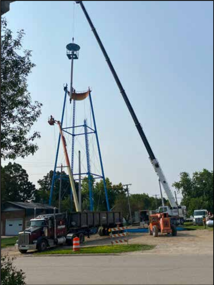
Taking down the water tower in Winger.
