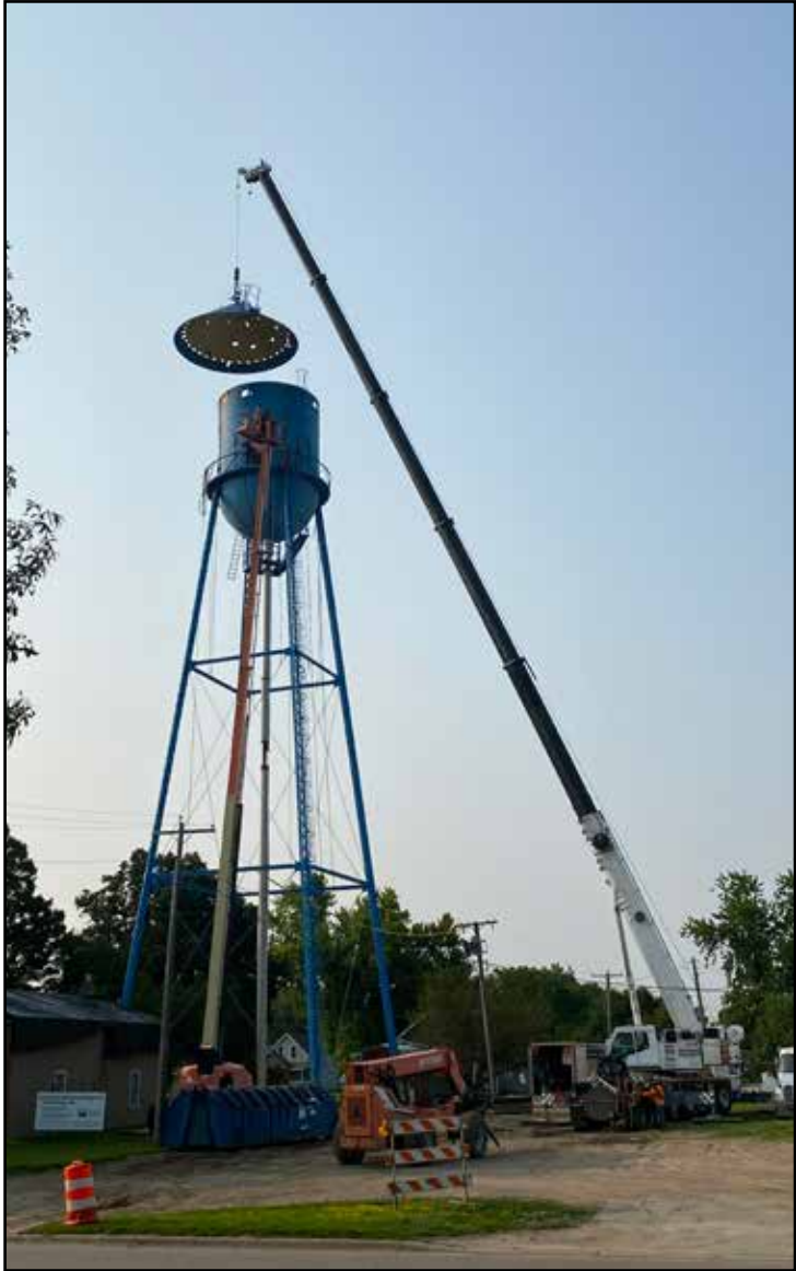
The roof is lifted off the water tower as demolition begins in Winger.
