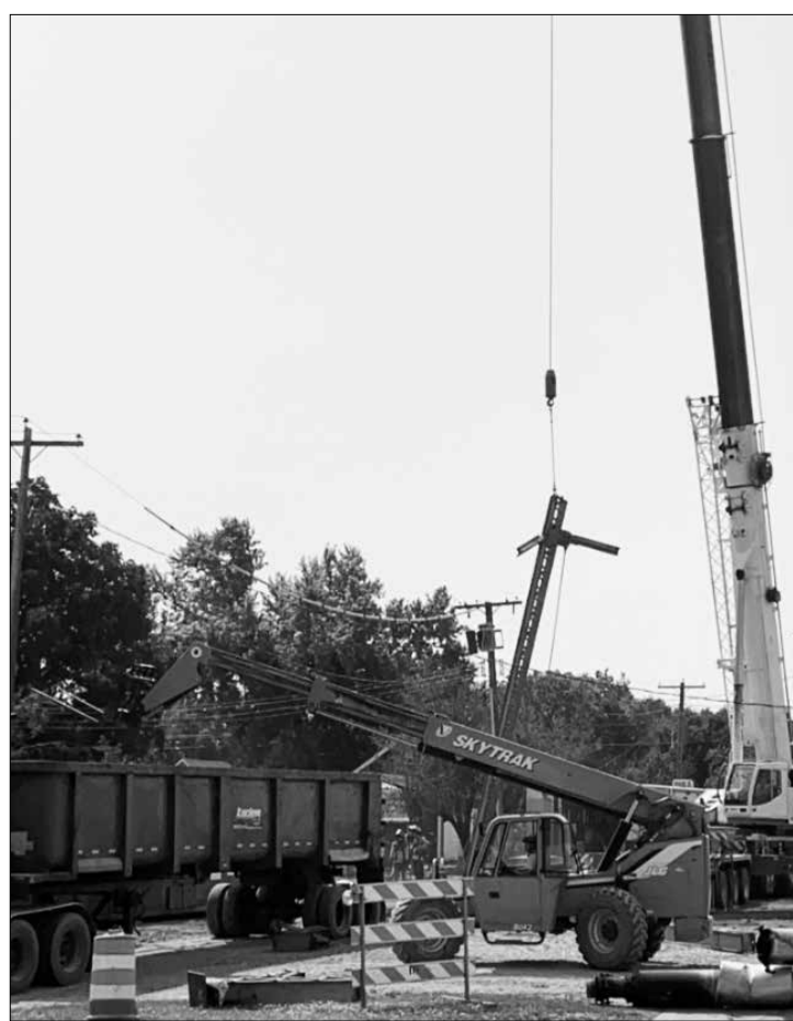
The last leg of the Winger water tower, which stood firm for 77 years was removed last Thursday.
