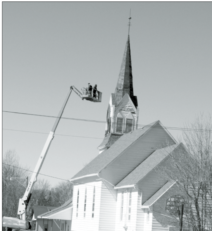
Along with the entire roof on Immanuel Lutheran Church in McIntosh, the steeple is getting new shingles. Here Dave Faldet's crew is working on the very tall structure last week.
