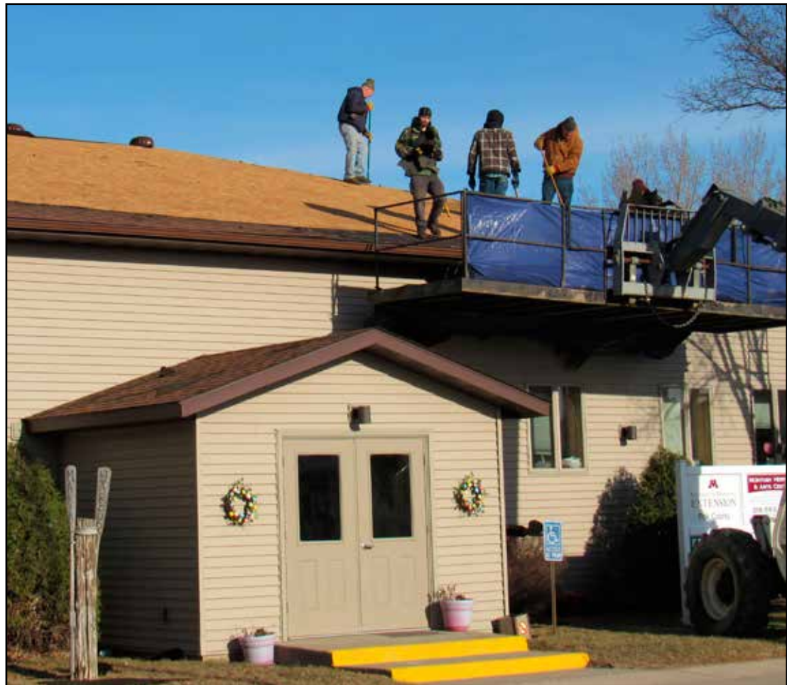
The Bjella Building, a City of McIntosh municipal building, received new shingles due to storm damage that occurred last summer. Dave Faldet and crew took advantage of our early Spring weather to tear off and replace the roof on the building. The project took them nearly a week, and the roof was completely reshingled. The Bjella Building was originally constructed in 1965 and served as offices for the City of McIntosh, among other services until 1989, when the new Community Center was constructed.
