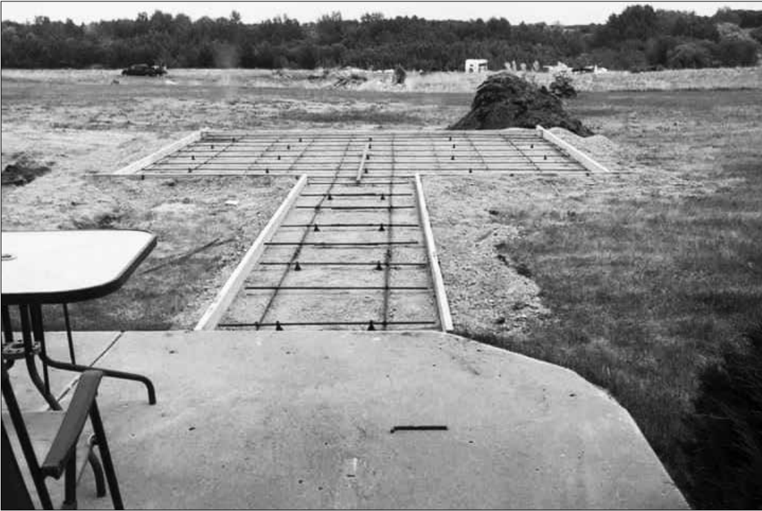
In July, the gazebo plans were made and the form was laid out at Poplar Meadows Senior Living.
