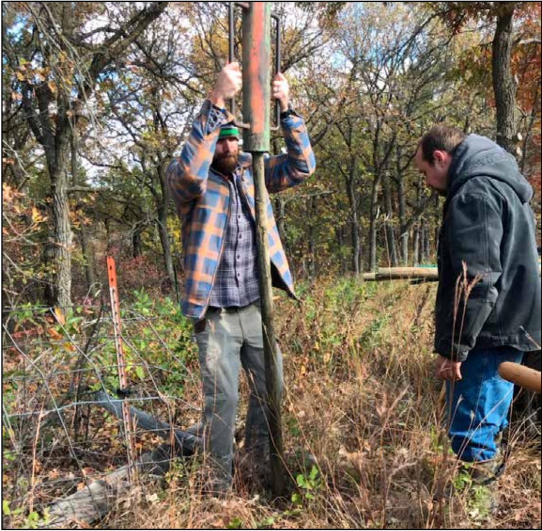
The Polar Beach Snowmobile Club recently spent a sunny day working on the Sleepy Hollow Snowmobile Trail, a trail that runs from McIntosh to Trail, MN. The Club cleaned up debris, widened some areas on the path and installed new signage along the trail. More work by the Club will continue on this trail, and others, throughout the fall. Pictured (l-r): Dominic Kringlen does the heavy lifting of pounding posts with Matt Thompson looking on in observation.
