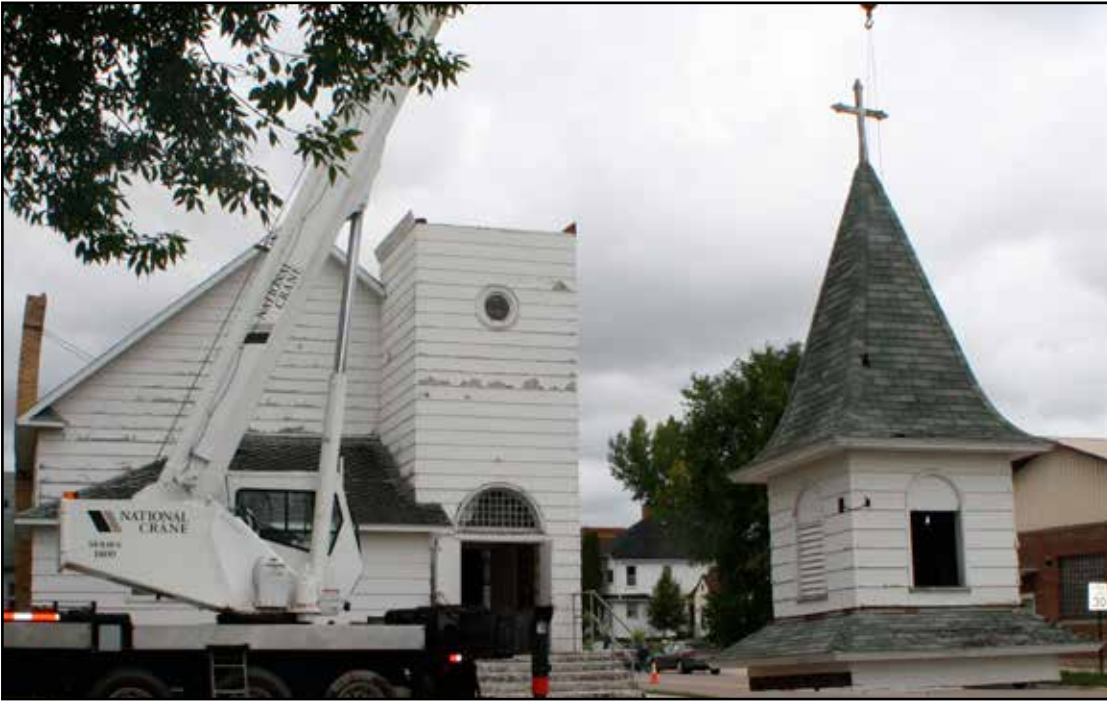
The steeple from Salem Church in McIntosh was taken down and relocated on Friday, September 11th.
