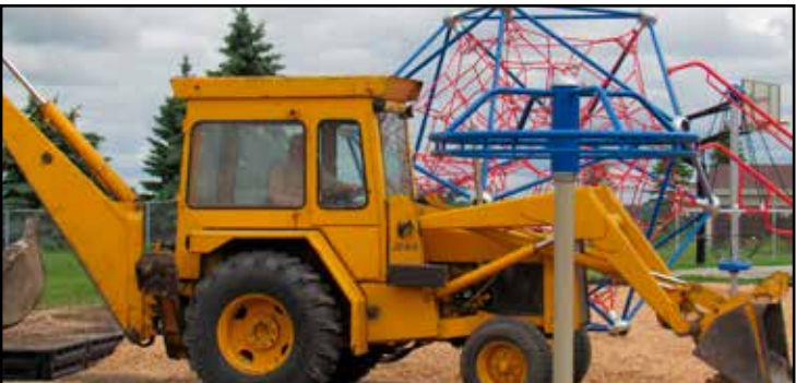
Volunteer, Joel Strom brings in the heavy equipment to help move and spread out the woodchips as the final phase of the Win-E-Mac playground is completed.
