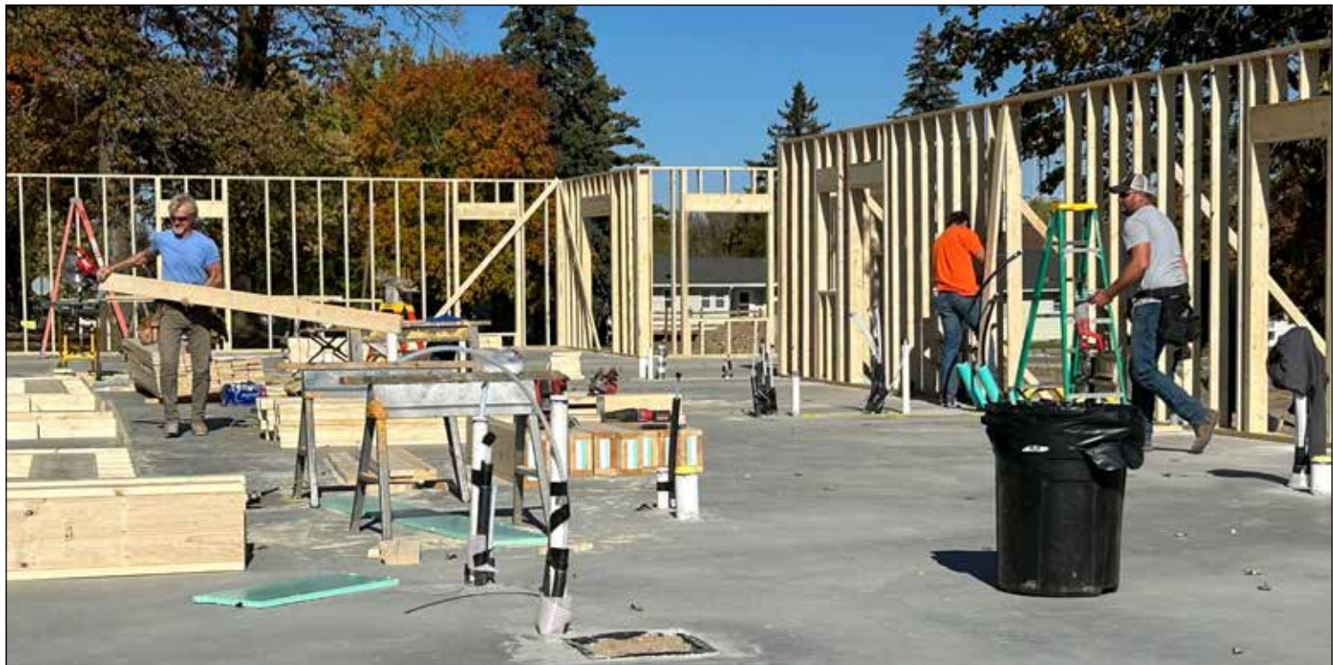
Progress in Clearbrook with the new duplex being built. The unit is located on the lot that was used for parking at the former Good Samaritan Center. That center has since been torn down with several loads of gravel being trucked in to the area. Gustafson and Goudge has this crew getting the walls up for the two unit addition to the town. Each unit will have a garage.
