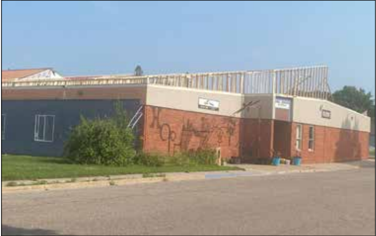
The roof is coming up at Clear Waters Life Center in Gonvick. Flat and semi flat roofs are a problem. This addition should solve the situation.
