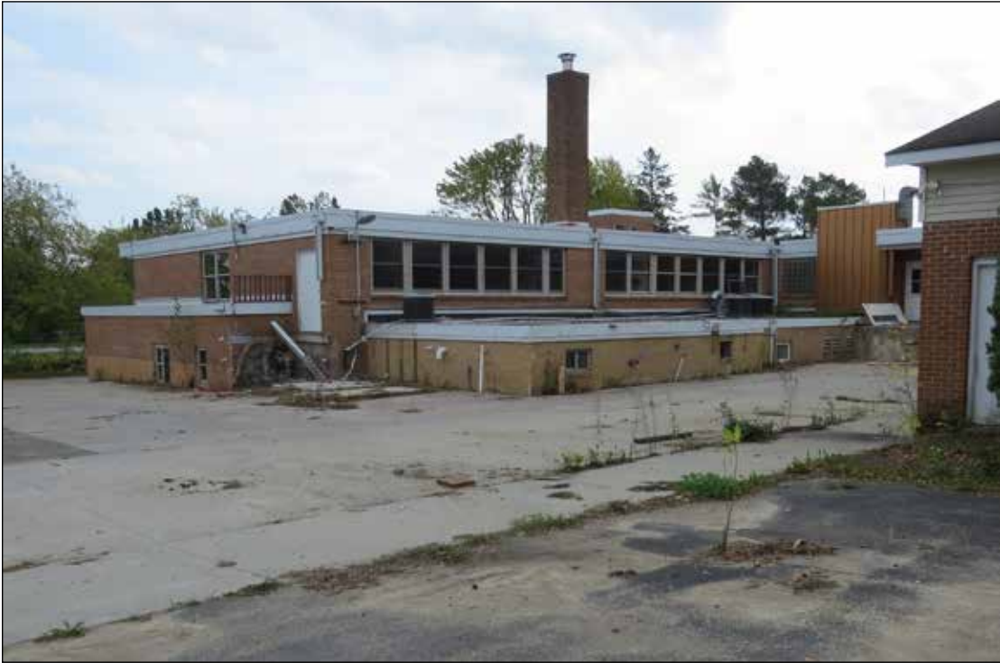
Good Samaritan Center is coming down to make way for new facilities.
