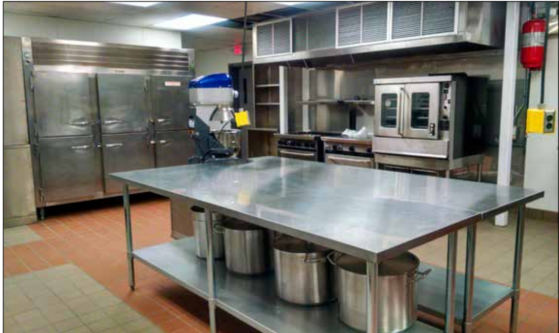
This is what is located in the kitchen facilities at the Clear Waters Life Center in Gonvick. It is in what was the old school office space and storage area.
