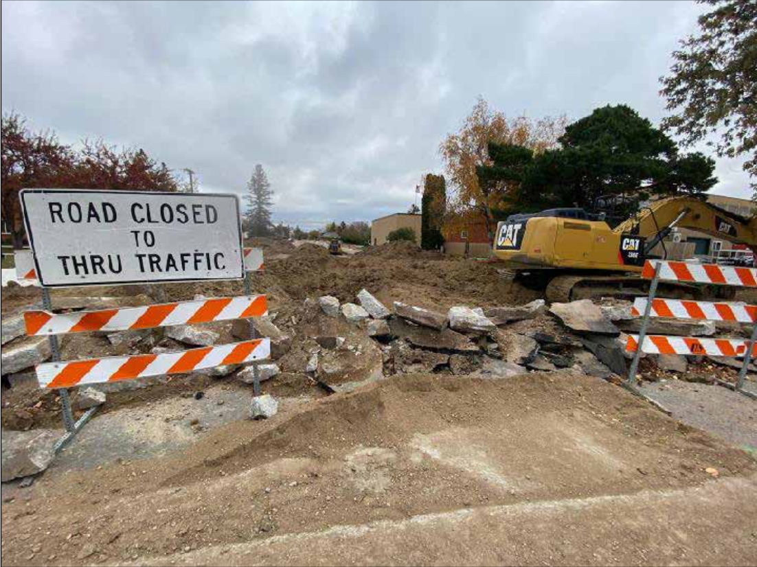
Change Order #7, which is a located between the old school and the Good Shepherd church had a pipe connection that needed fixing. That section has been torn up and the cost will be $100,000 that would not be paid by the city but with grant money.
