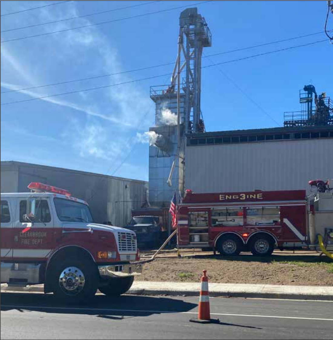
A fire at the Riviana rice plant in Clearbrook started about 1:30 pm on Tuesday, September 27. Julie Wraa, General Manager, explained that fire was contained to the dryer unit and damage was limited to that structure only. They do not know what caused the fire. They are currently investigating the cause and extent of the damage to the dryer unit. They are taking steps to minimize the disruption to their operations. There was no other damage to buildings nearby. Wraa stated that the two other dryers are still operating. All employees were evacuated from the nearby area as a precaution. No injuries were reported. The Clearbrook Fire Department responded to the fire. An ambulance and Clearwater County Sheriff Deputy were also on site.
