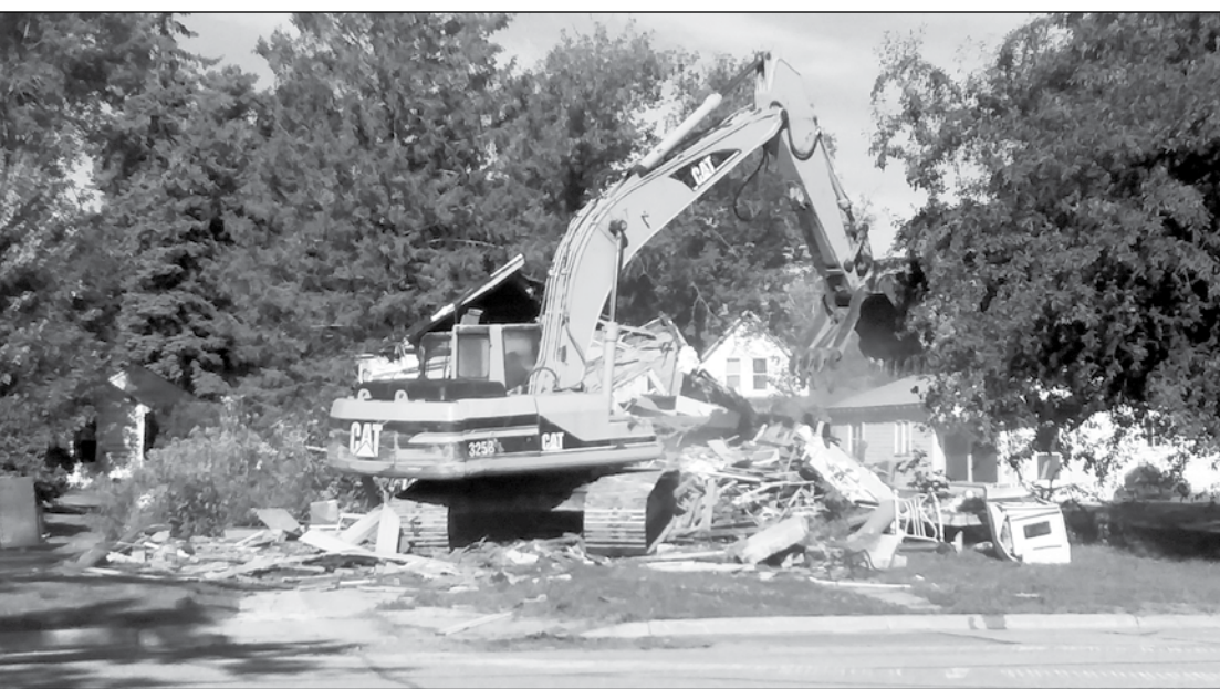
Jeff Jorgenson was back in Gonvick taking down a house on the east end of town that belonged to several people including Brenda Skime and before that time Mildred and Soren Birkeland. He was on his seventh load to the land fill. Photo by Jeff Blaele
