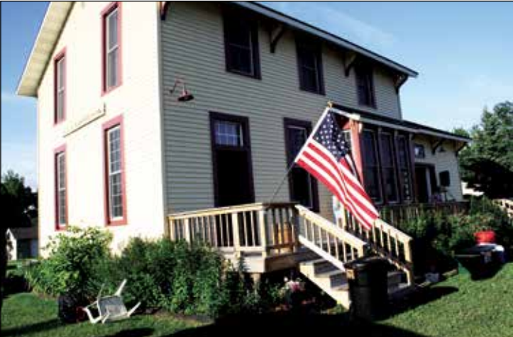
Restored Clearbrook Trail Depot 2017.
