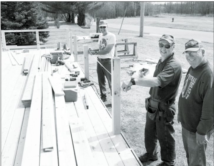
New decking has been put around the front of the old depot in Clearbrook. Working on the project are from left to right: Russell Lembke, Brad Borene and Glen Trembath.
