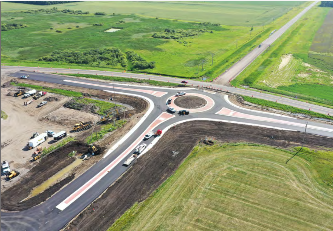
Roundabout near completion south of Thief River Falls.
